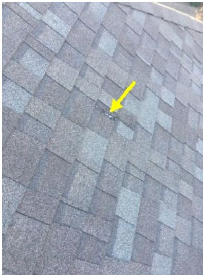
Damaged Shingles
