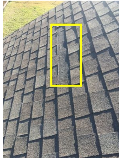
Missing shingles
